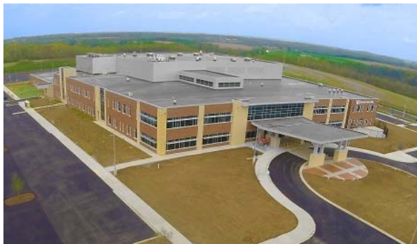
Construction is now complete on a new VA health care center in Butler, Pa.
