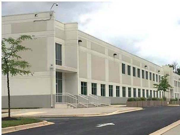
The Washington Metropolitan Area Transit Authority purchased the property located at 10201 Good Luck Road in Lanham, Md.
